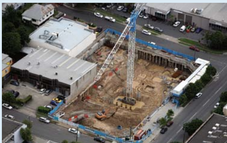
CONSTRUCTION works on the $38.5M AUSENCO Centre at 144 Montague Road, South Brisbane for the Ray White Invest Montague Road Property Trust, began in late August 2008, with completion due by December this year. Jeff Miller and his site crew powered through the retention system and completed the basement ground slab prior to Christmas.
